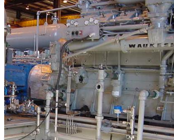
2,000 HP JGT/6 Ariel Compressor with Waukesha 9390 Engine Drive
